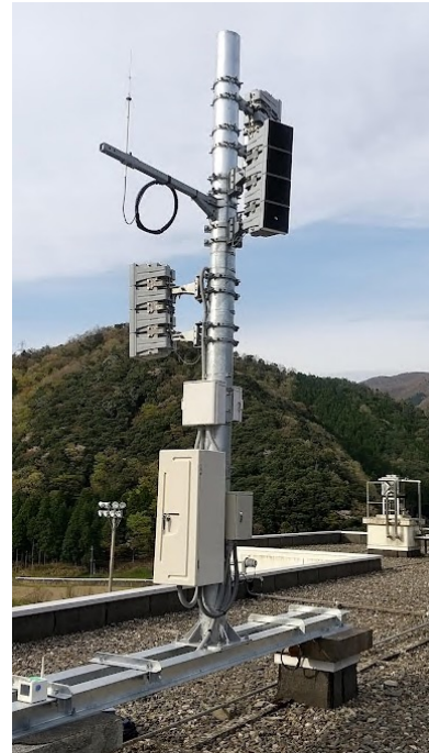
Disaster mitigation communication system Broadcasting device
